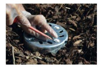
Once the post is rotated into the correct position (refer to the site plan!), the clamping unit is screwed in place. Tighten the screws using a ratchet wrench and a 13 mm socket.
