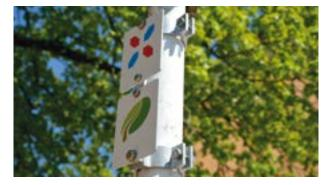
The waymarking plaque should be mounted on the post at an appropriate height (approximately 2 meters). If needed, arrows are manually added to the waymarking plaque before affixing it to the post (see Chapter 1.4.5).
