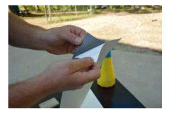
placed on the welded seam, as it may detach there. Leave a margin of about 1 to 2 mm around the film to prevent it from being torn off.
